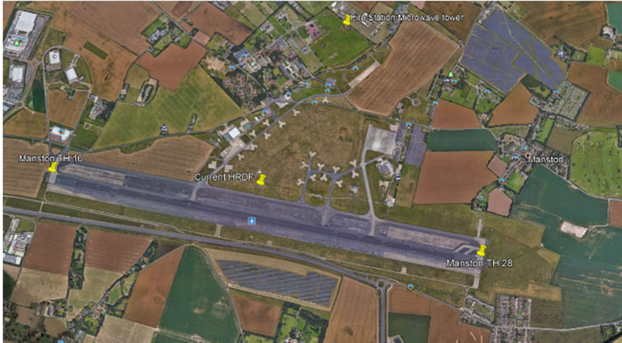
Figure 12 - HRDF Fire Station Microwave tower location
